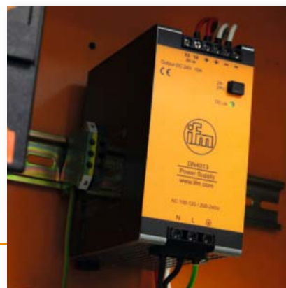
A small but useful detail: All 24 V switched-mode power supplies are equipped with double terminals. This simplifies wiring and provides more clarity in the control cabinet.
